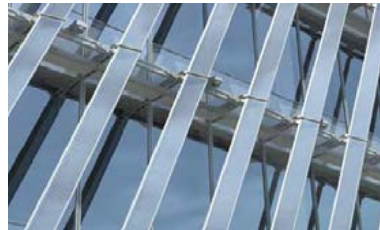
▲ tower sun shading detail
