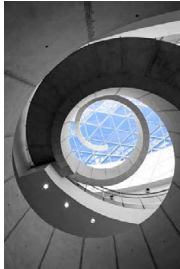
▲ helical staircase detail
