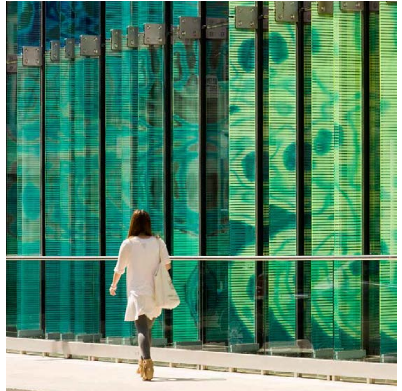
▲ façade detail, outpatient department
