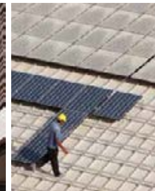
▲ high performance roof
