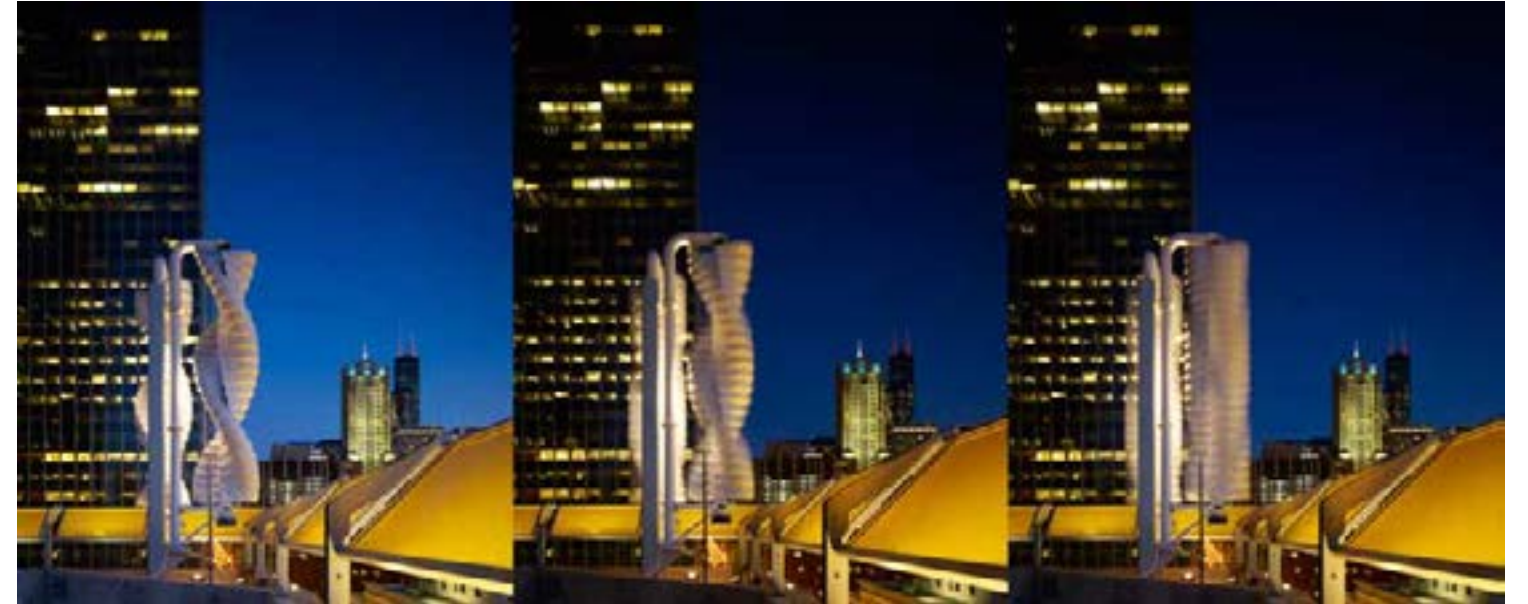
▲ wind turbine detail
