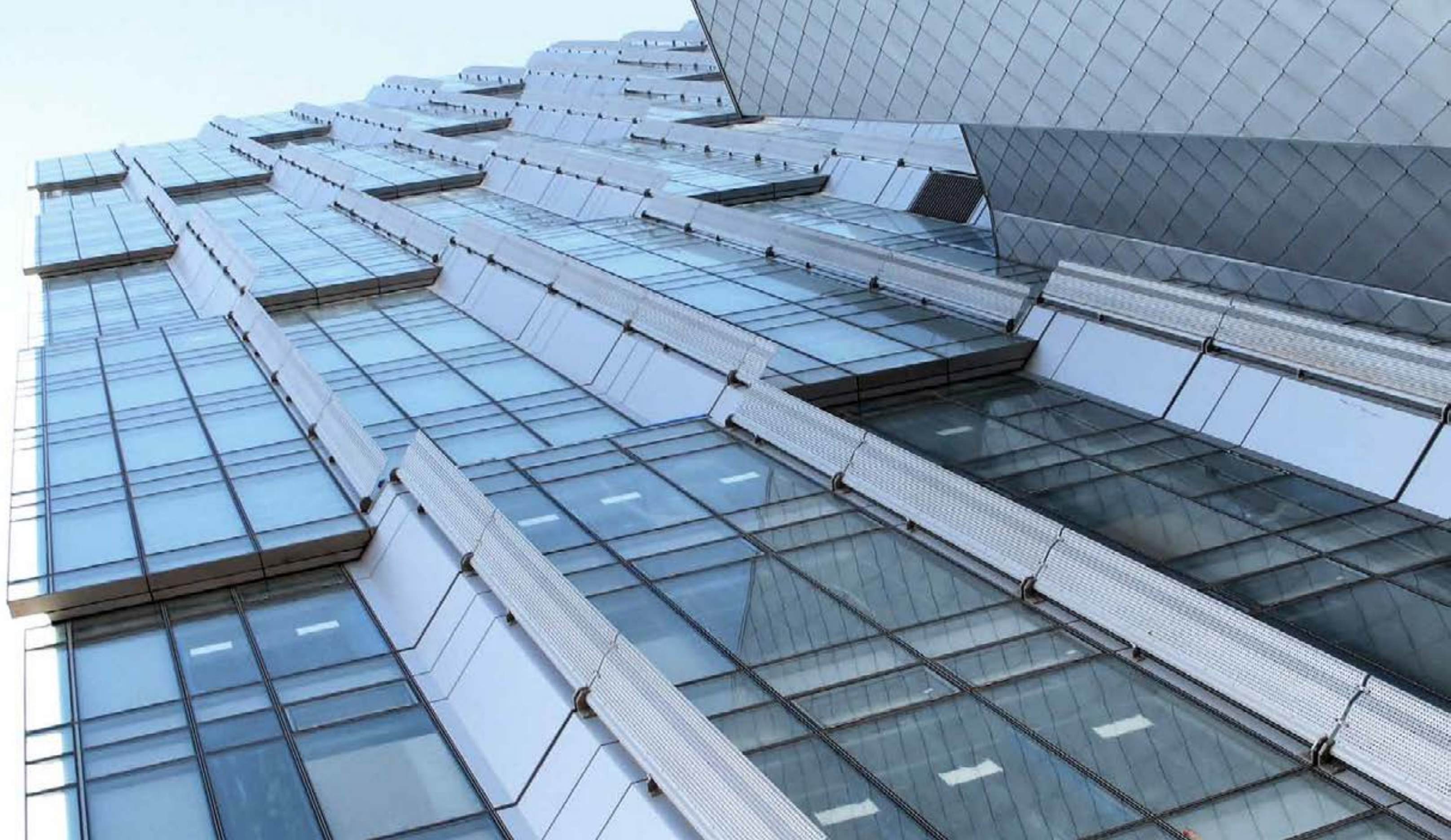
▼ north facade detail
