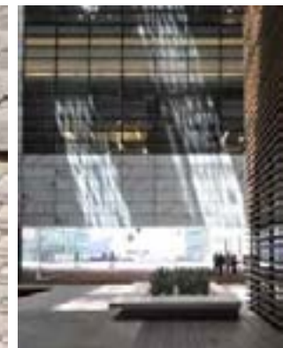
▲ passively cooled courtyards
