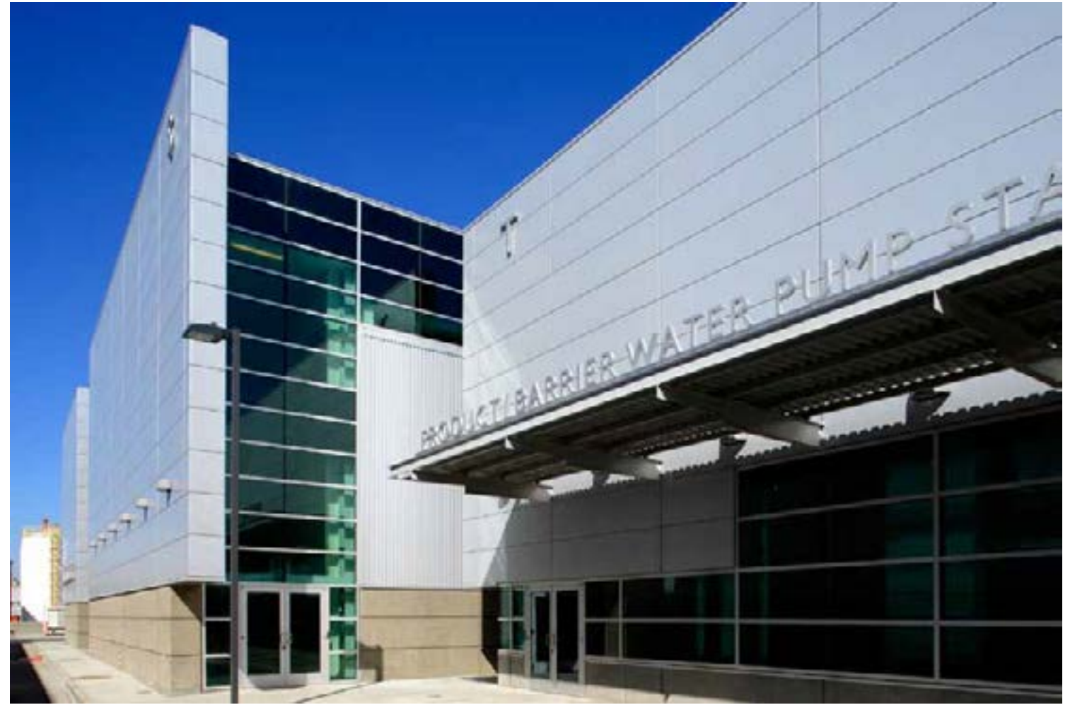
▲ pump station, west elevation
