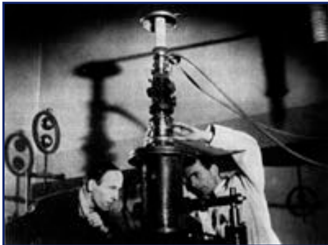
Electron microscope built by Ruska and Knoll in Berlin in the 1930s.
